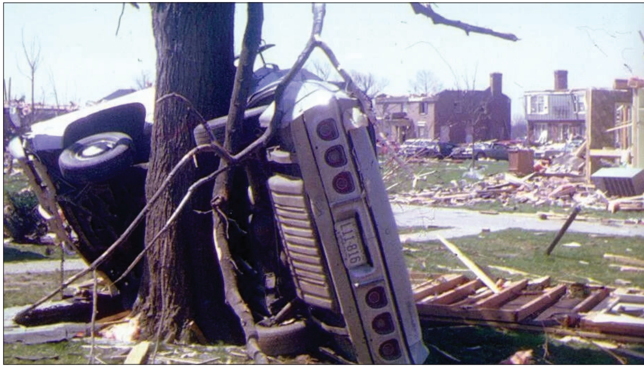
Destruction from the 1974 tornado outbreak that caused severe damage and loss of life in Meade County. Friday, April 3, is the 52nd anniversary of the tragedy in Kentucky.
