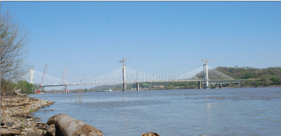
New Don Welge Memorial Bridge Wide View
