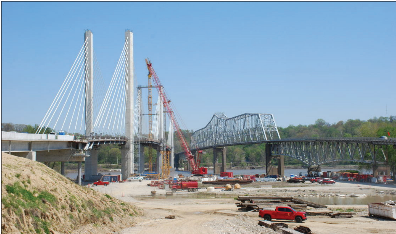
New Don Welge Memorial Bridge construction equipment.
