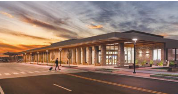
Barkley Regional Airport Photo by Eric Mueller
