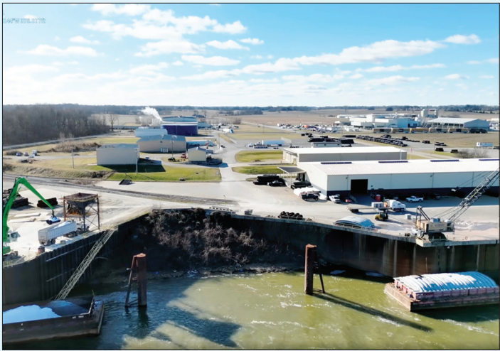
“A big milestone at the Henderson County Riverport Authority today. For the first time, we unloaded two barges at the same time. Our new Sennebogen material handler unloaded fertilizer while our 125-ton American crane handled a barge of aluminum.”-Henderson County Riverport Authority. Photo sourced from HCRA LinkedIn post.
