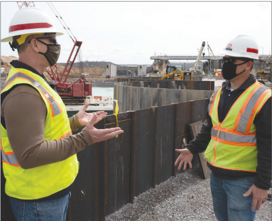
Barney Schulte (Left), lead engineer for the Kentucky Lock Addition Project, confers with Jody Robinson, Contract Team lead at Western Kentucky Area Office, while standing on top of the completed cofferdam at the Kentucky Lock Addition Project March 22, 2021 on the Tennessee River in Grand Rivers, Kentucky. The U.S. Army Corps of Engineers Nashville District is constructing a new 110-foot by 1,200-foot navigation lock at the Tennessee Valley Authority project.
