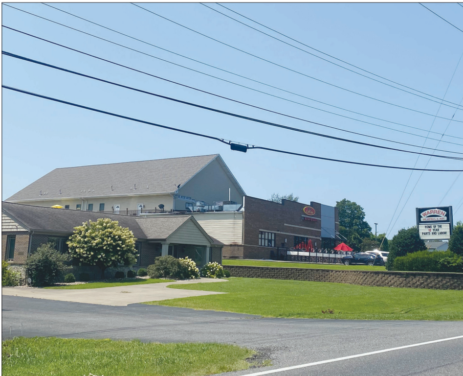
Warren Heating & Air owner Steve Warren launched his one-man operation in 1983 serving the community's heating and air conditioning needs. Today his firm has grown to 14 highly educated and trained service technicians delivering excellent, year round customer service to homeowners and businesses across the region.
